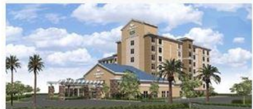
Homewood Suites by Hilton Orlando Convention Center South
